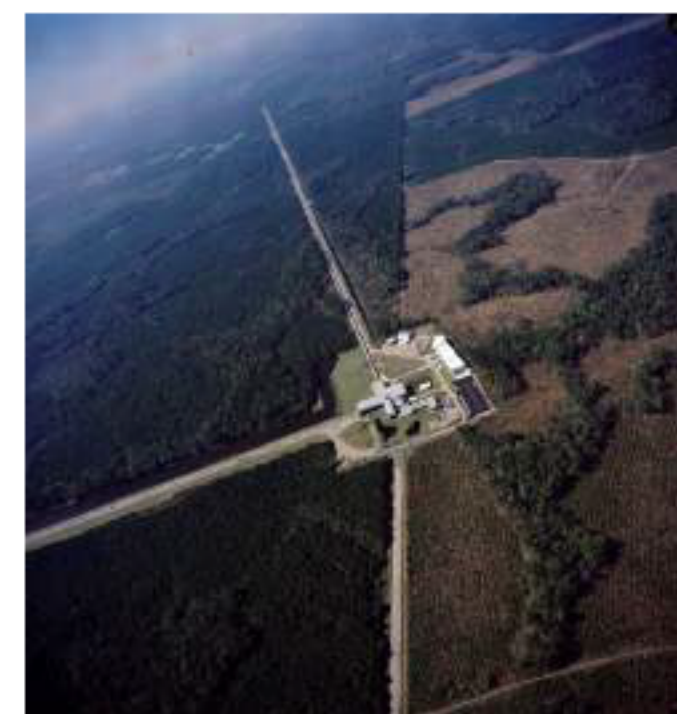
An aerial view of the LIGO detector in Louisiana. Courtesy of LIGO Laboratory.
